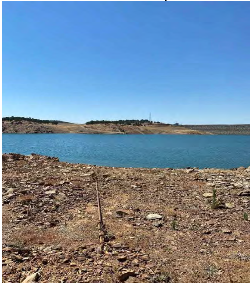
Shoreline Deadman Anchor – West Bay 760' Water Level
