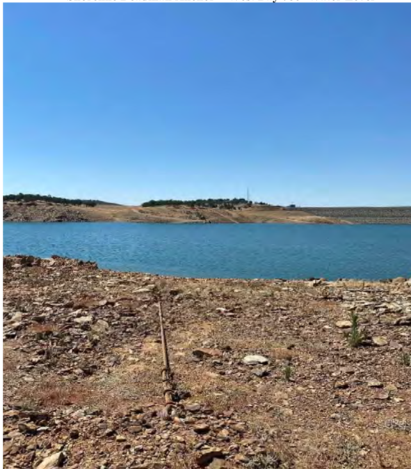
Shoreline Deadman Anchor – West Bay 760' Water Level
